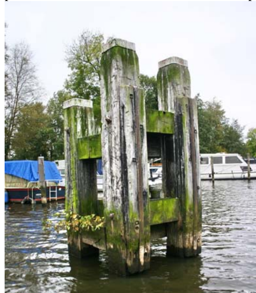
Figure 1: Mooring pole Zwartsluis/Netherlands
