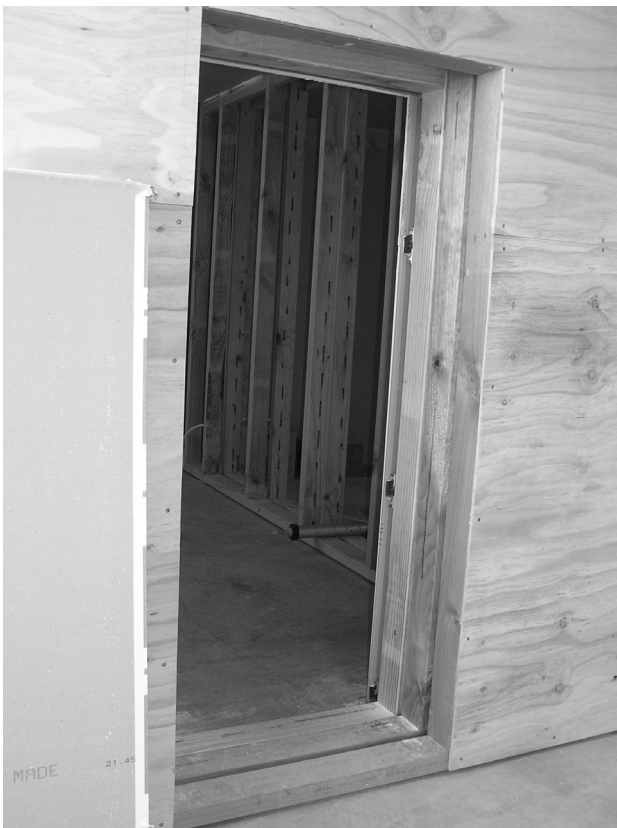
Figure 1. Acoustically-isolated test chamber under construction for the Multi-Function Timber Joints Project.
