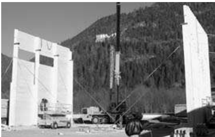
Figure 3. Cross-laminated industrial building under construction.
