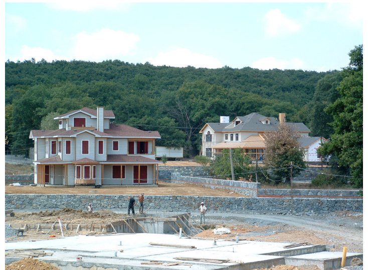
Figure 5: Examples of timber frame construction in Turkey
