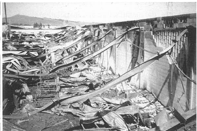
Figure 5. Unprotected steel portal frame warehouse after a fire (15).
