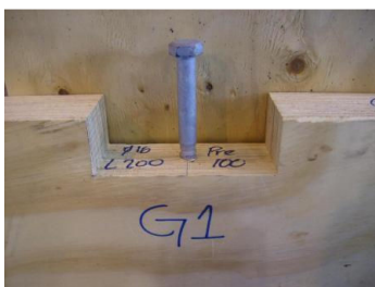
Figure 2. Notched coach screw connection detail
