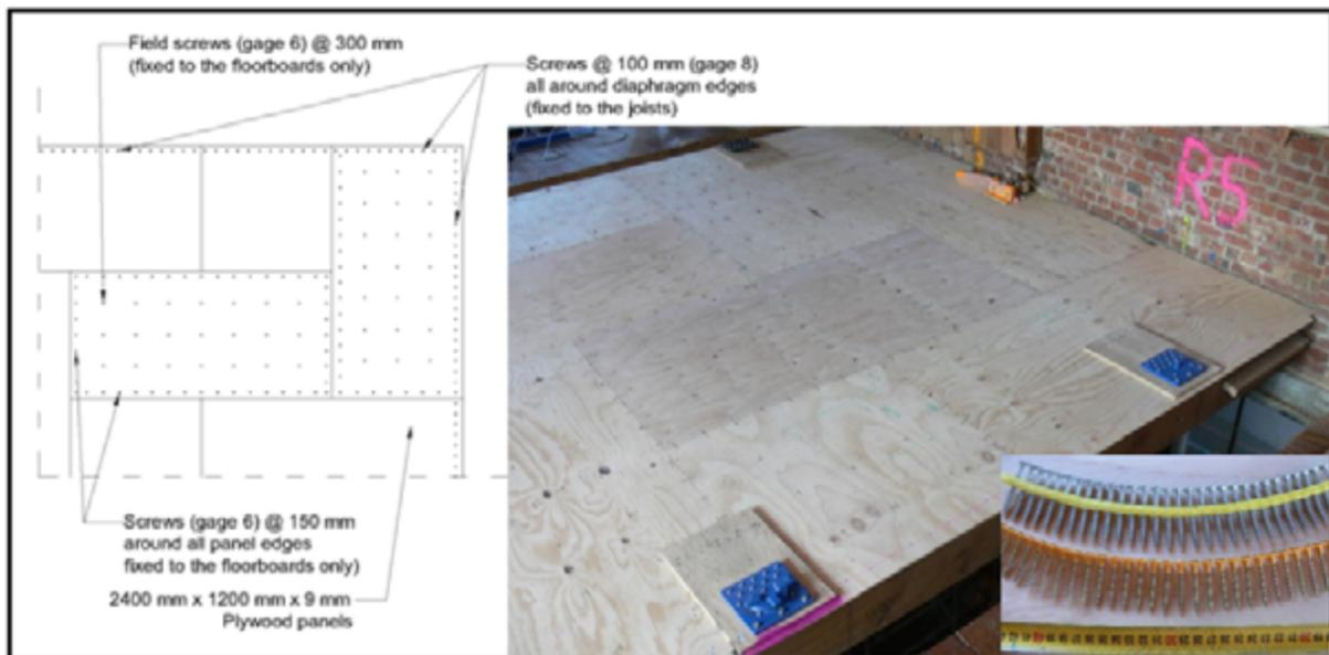
Fig. 4 Plywood overlay disposition
