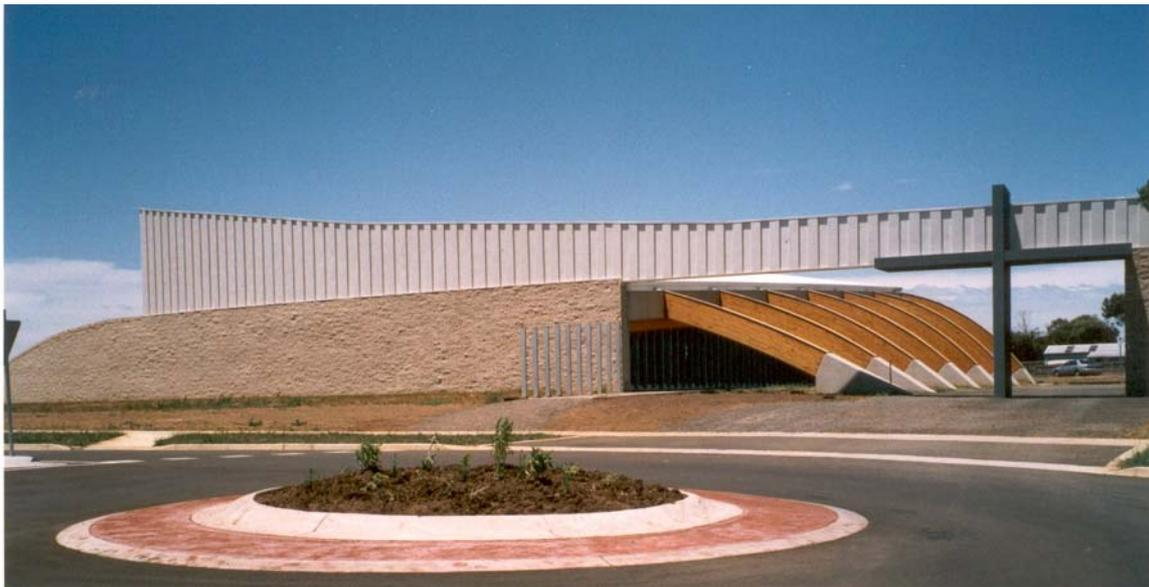
Entry to the site from the north west was through a large curved masonry block wall and cross that creates a view of seven individually curved laminated beams which were perpendicular to the length of the building. The concrete raised beam connections create a ceremonial walkway adjoining a timber sleeper pathway to the entry at the opposite south east end of the building.
