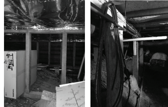
Figure 4-6 Examples of Unbraced Foundations
