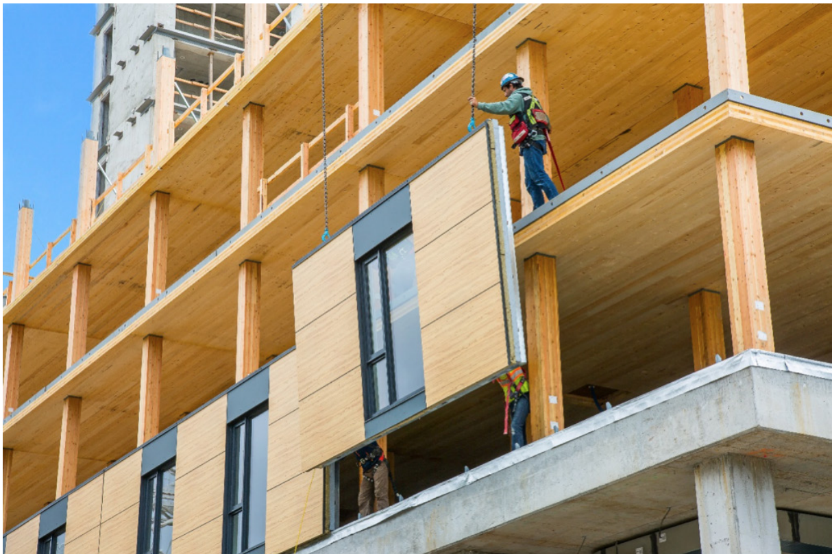
Figure 8: Prefabricated façade installation. Courtesy of Seagate Structures.
