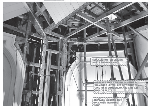
Figure 10: Example investigations and repairs
