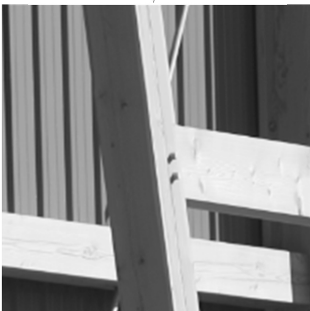
Figure 5. Oak pegged mortise and tenon connection. (Source: 2011 Canadian Timber Frames Limited)
