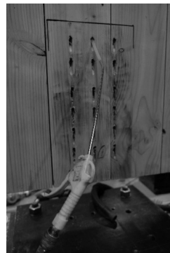
C - Blowing out of dust
