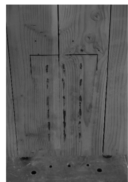
F - Finished repair ready for new fasteners
