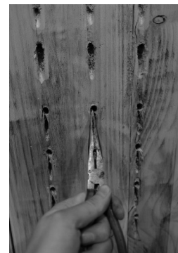
B - Removal of loose fibres with pliers
