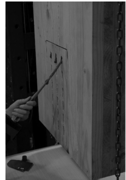
D - Injecting of epoxy
