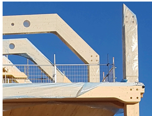
Figure 8: On site picture. Direct timber connection.
