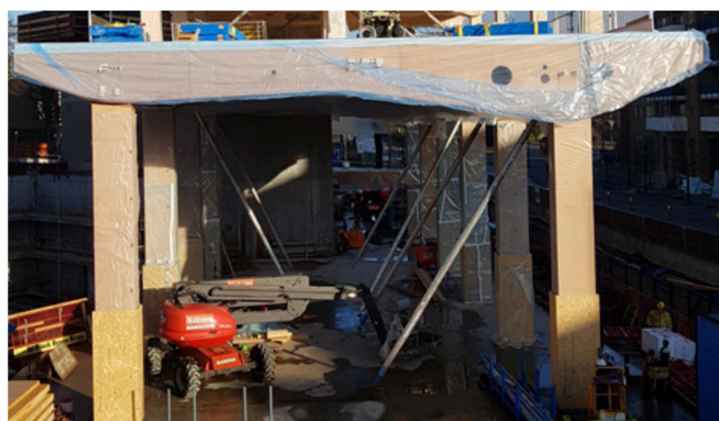
Figure 7: LVL beech beams and columns. LVL insertions.
