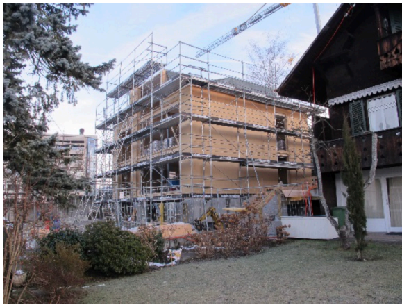
Figure 26: Building site of a multi-storey building Thun, Switzerland.
