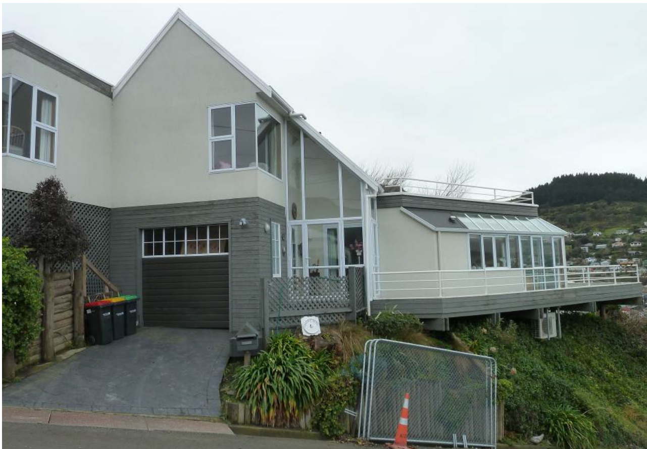
Figure 7. House on sloping site with horizontal and vertical irregularities and differing foundation types.
