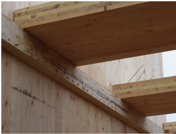
Figure 8: Floor to ledger connection at the core.
