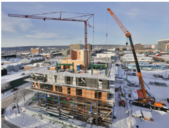
Figure 6: CLT core installation in progress.
