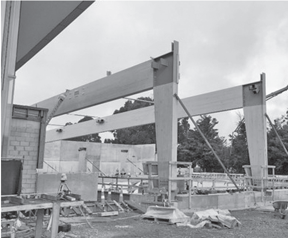
Figure 5: Portal Frame Installation
