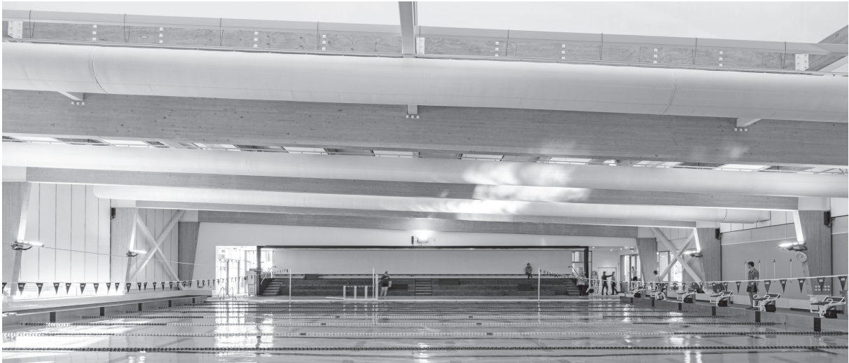
Figure 1: Selwyn Aquatic Centre Extension
