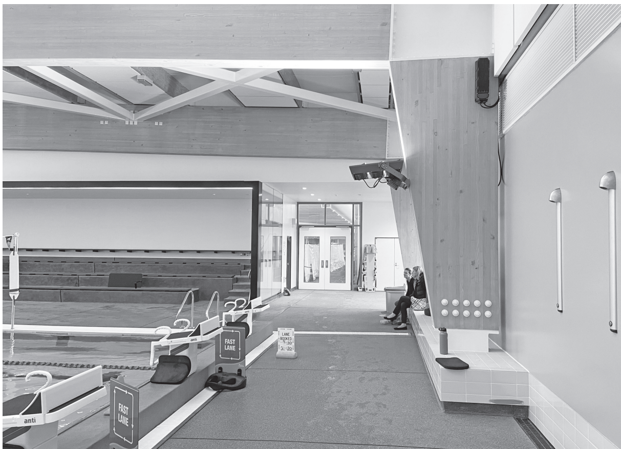
Figure 7: Portal Base Connection
