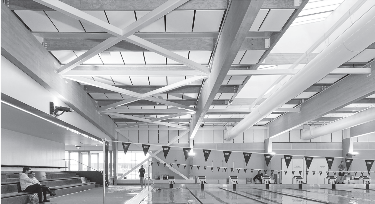
Figure 6: SHS Braced Bay
