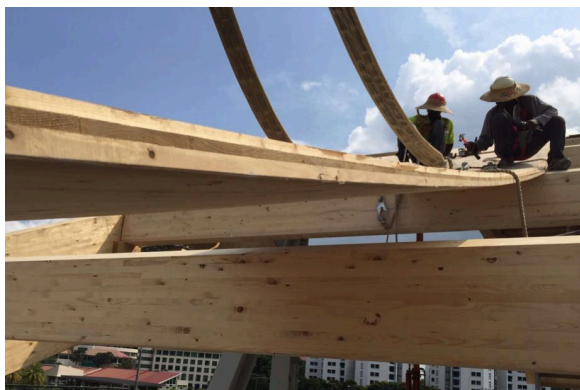
Figure 14: CLT stiff diaphragm on the roof.
