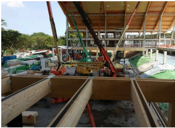
Figure 19: Main glulam coupled beams on the exterior façade.
