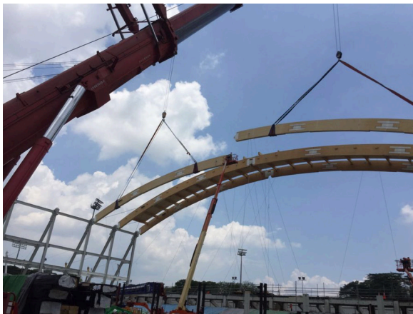
Figure 16: Launching of arches.
