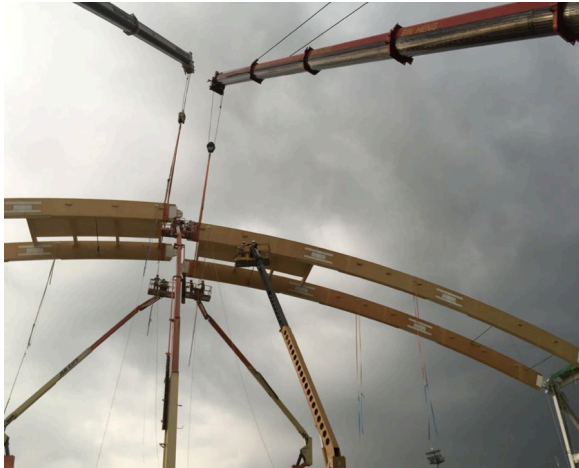
Figure 16: Launching of arches.
