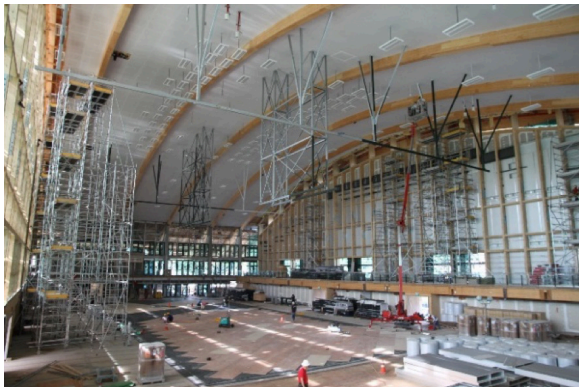
Figure 19: Main glulam coupled beams on the exterior façade.
