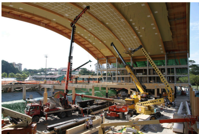
Figure 18: Phases of the erection sequence of the interior stories.
