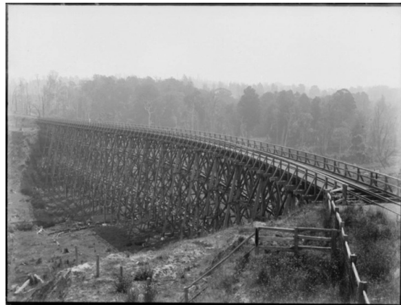
Figure 2 - First Ormondville railway viaduct in southern Hawke's Bay (Williams, 1891-1983)
