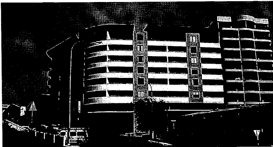
Gulf View Towers, Auckland, 5 stories, all light weight timber construction
