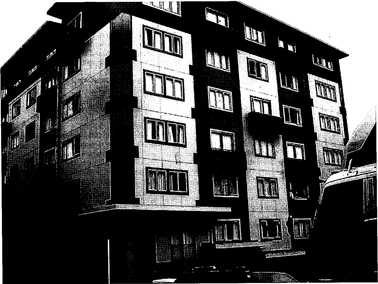
Martin square apartments, 6 storeys, predominantly light weight timber construction
