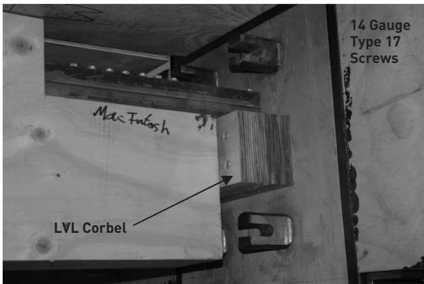
**Figure 2. Hanging beam/floor joist connections.**
