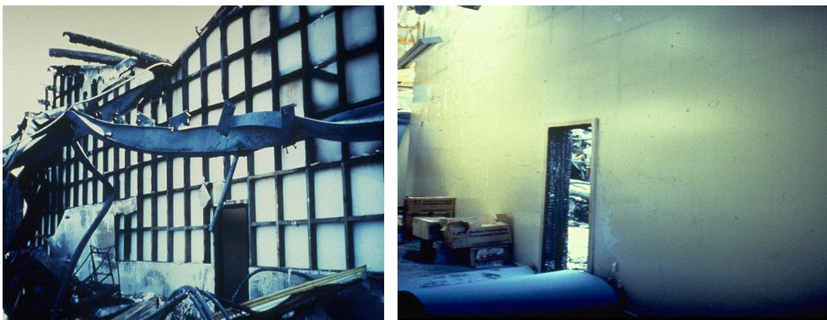
**Figure 4:** Timber framed partition lined with gypsum plasterboard after a building fire
