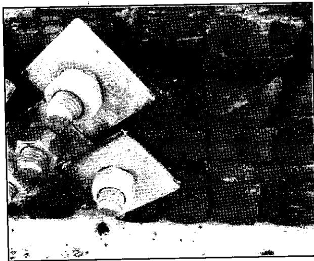
Figure 9 Failure mode of W-S-W bolted connections
