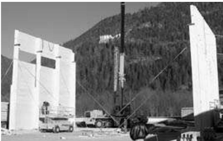
Figure 3. Cross-laminated industrial building under construction.
