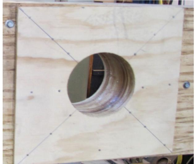
**Figure 4. Reinforcing with plywood.**
