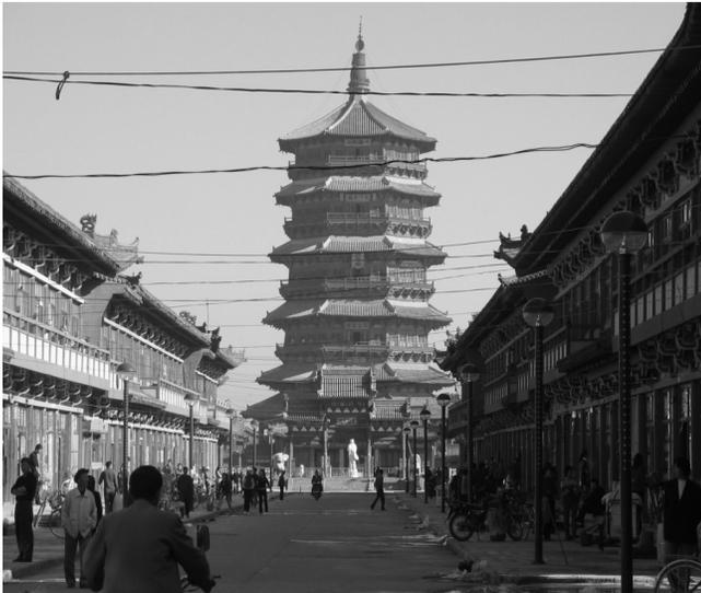
The timber pagoda at Ying Province was completed in the year 1056. It is octagonal in plan view. It is composed of five stories (entirely of wood) and is approximately 67 metres above ground level. The external of the pagoda showed a subtle taper of the structure from the base to the top.
