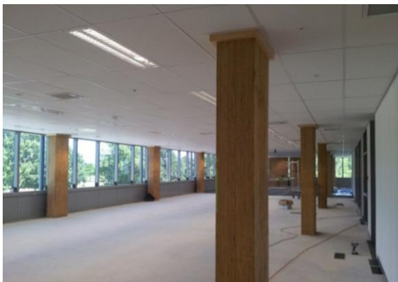
Figure 12: Wood columns exposed.
