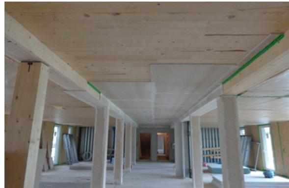
Figure 14: Wood ceiling, beams and columns during process of encapsulation with fire-resistant board.
