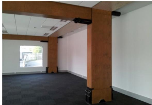
Figure 13: Wood columns and beams exposed, also post-tensioning anchorages and dissipation devices.
