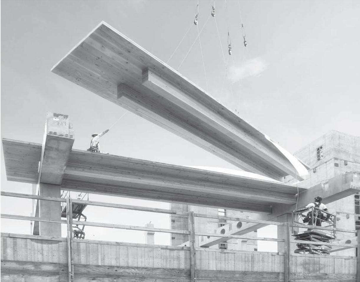
Figure 4: Timber floor panel placement
