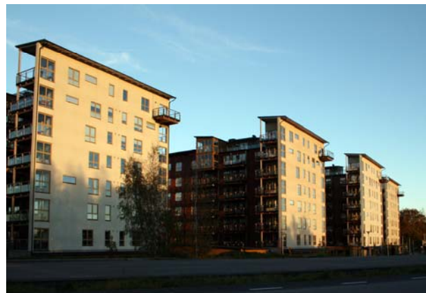
Image 8: 8 Storey residential buildings in Växjö Sweden
