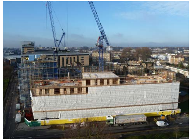
Image 6: Installation Bridport House
